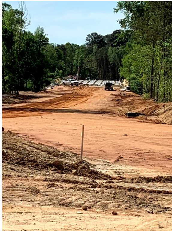
Figure 14 - Bridge construction over Wagner Creek
